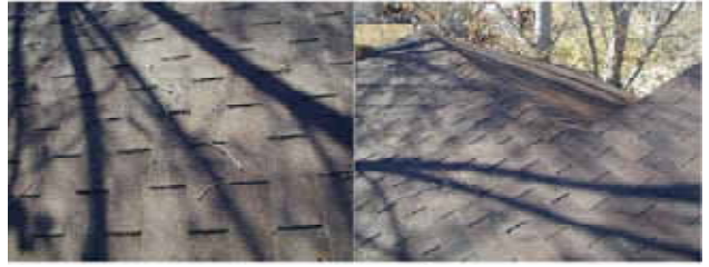
Porch, shed and SW corner of roof
