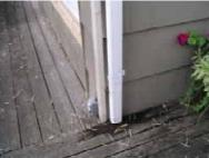
upgrade the gutters with debris covers. 2) Downspout at guest house should be extend to drain away from deck and foundation.
